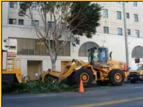
Tree trimming & street light repair
